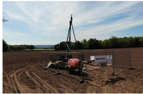
Core percussion rig used for drilling boreholes
