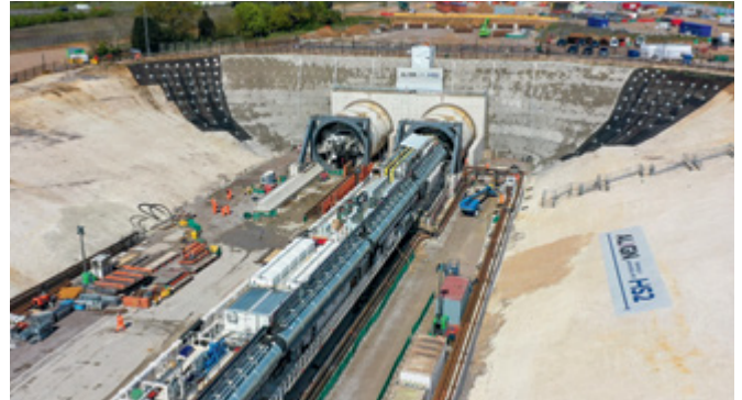
The Chiltern Tunnel South Portal site is the home of two tunnel boring machines and the main site for the construction of the Colne Valley viaduct.
